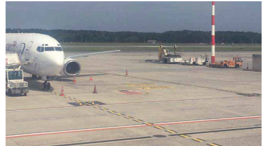
Malpensa 2000 Airport Varese - Italy
